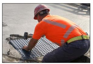
3. Place the Step-Safe® tiles into the freshly poured concrete, evenly in lines parallel to existing edge conditions, or as directed by the architect or engineers drawing. Leave a minimum 1/8" gap between adjacent tiles on all sides to accommodate expansion.
